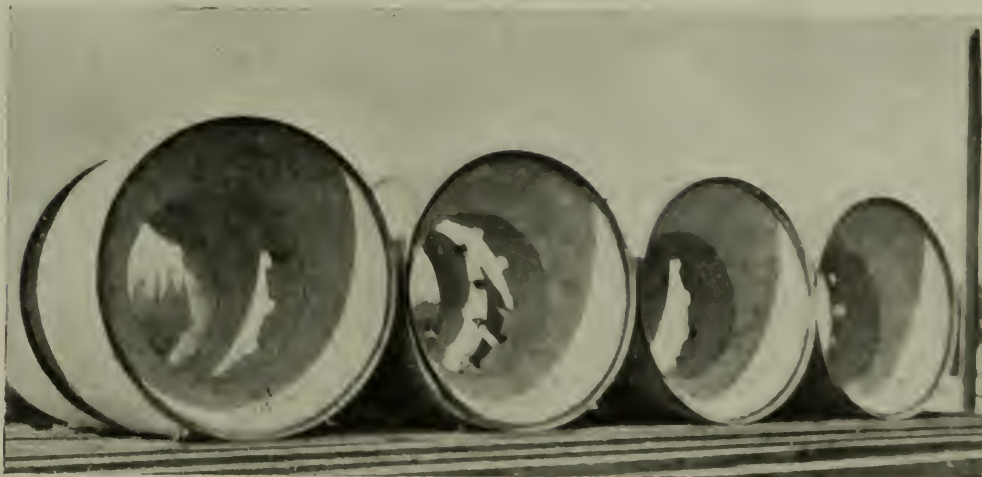
NEW HARBOUR WORKS AT VANCOUVER CYLINDER SHOES. (See p. 660.)
